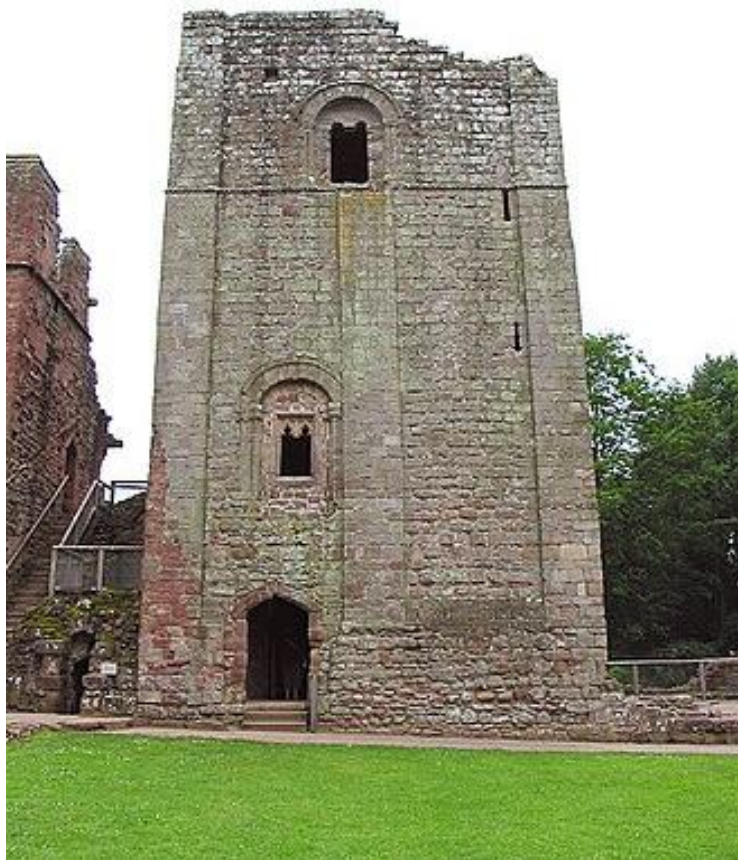
The Norman square keep of Goodrich Castle in Herefordshire in England, with the original first-floor doorway still visible above its later replacement (CC BY-SA 2.0)
