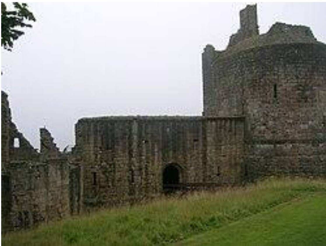
Ravenscraig Castle in Scotland, showing its curved, low-profile fortifications designed to resist cannon fire (© user:kilburn)
