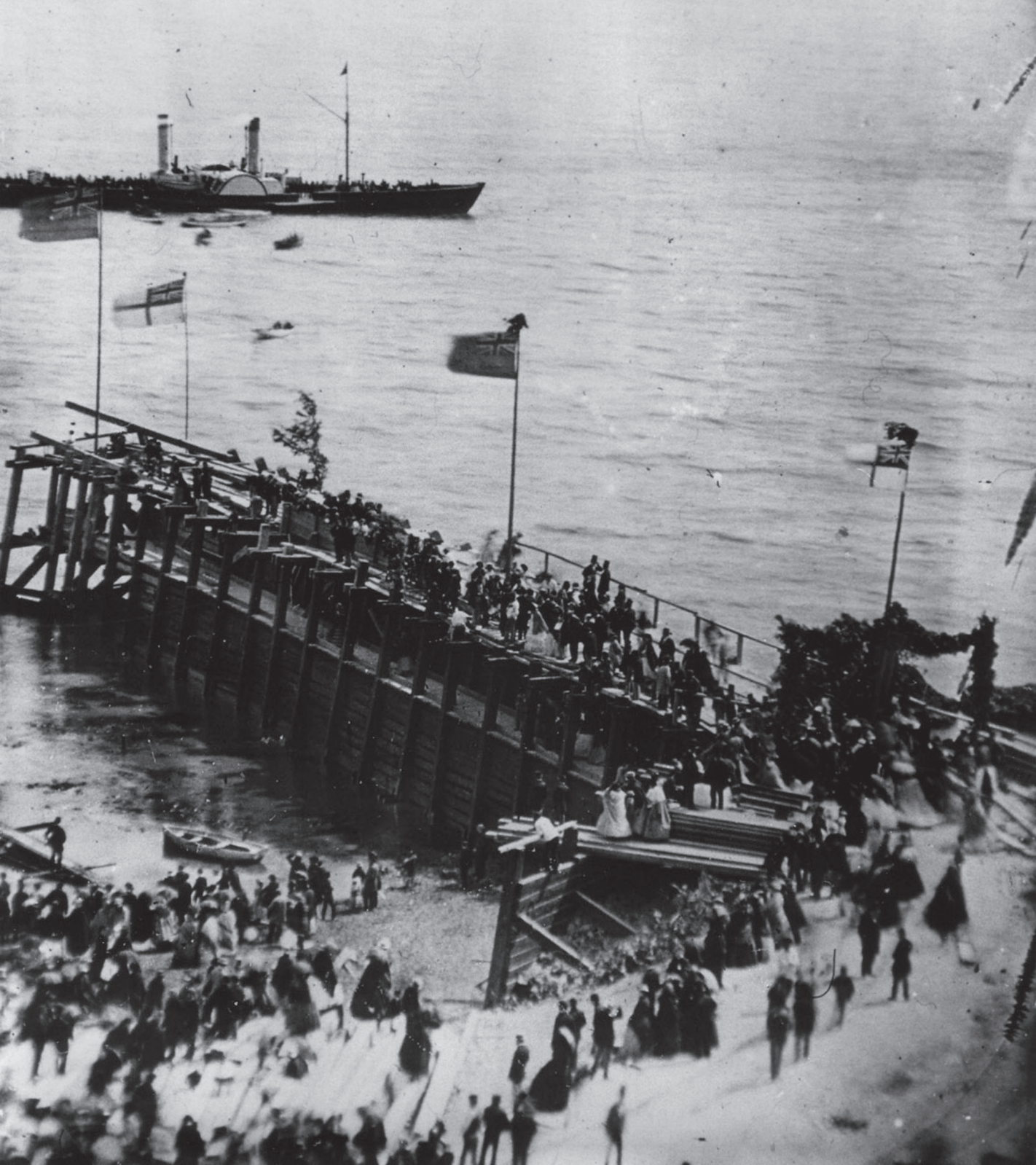
The very incomplete western breakwater of the refuge harbour on 29th June 1863. On that day, even though only around 100 yards of the breakwater was in place, the Harbour Company decided to open it to visiting steamers. In this view, in conditions of low water, the 170-foot, twin-funnelled paddle steamer 'Chancellor' is anchored out in the Bay and can be seen landing passengers by means of small boats. Notice the celebratory arch of foliage at the entrance to the breakwater and the many flags. Two days later the same paddle steamer called again and was brought alongside the pier on a falling tide. When, several hours later, she went to move astern to depart, it was discovered that her bow had grounded on rock. That night, as the tide came in, her fore compartment flooded. Later, strong winds blew up and, in a heavy swell, the vessel broke her moorings and her stern turned broadside on to the beach, the hull eventually breaking in two. It was an ill omen.
