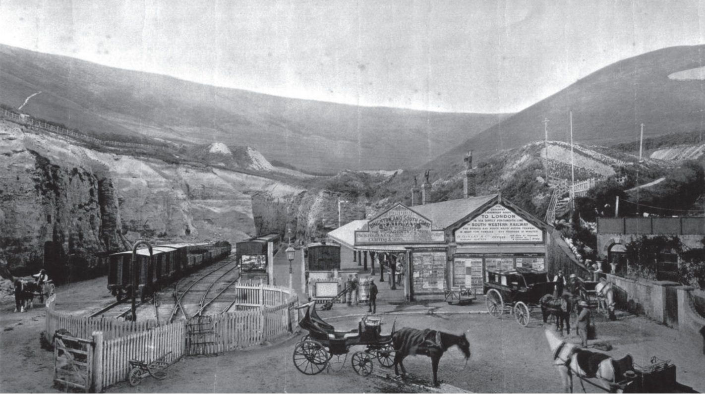
Ventnor station in the first decade or so of its existence, with an omnibus and a private carriage awaiting custom.
