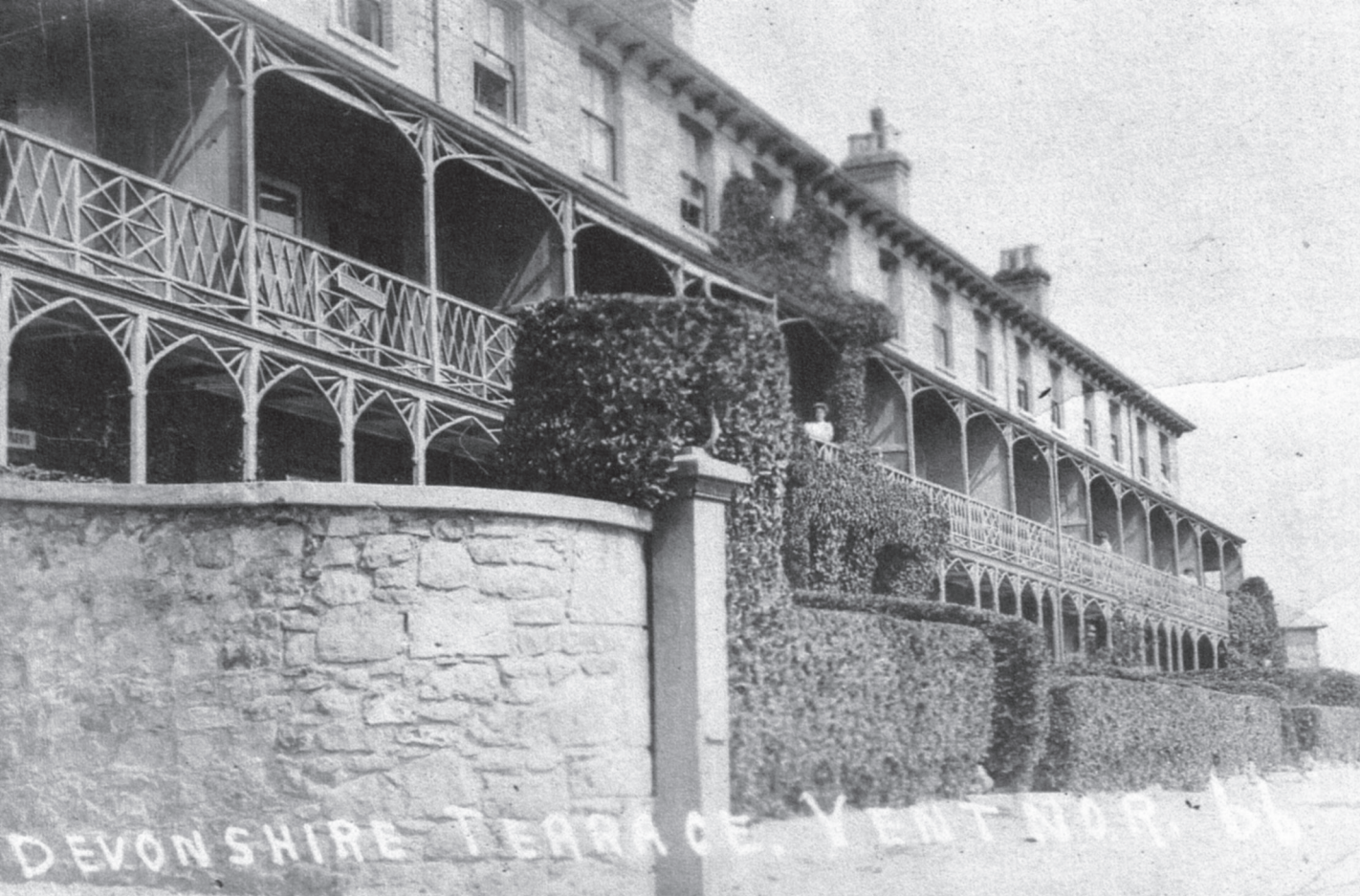
Devonshire Terrace with its elaborate wooden balustrading, a model of uniformity of stylistic treatment
